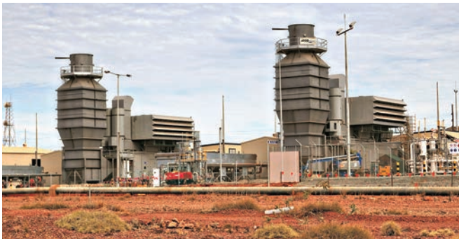
EXHAUST SILENCING SYSTEM FOR 2 X GE LM6000
