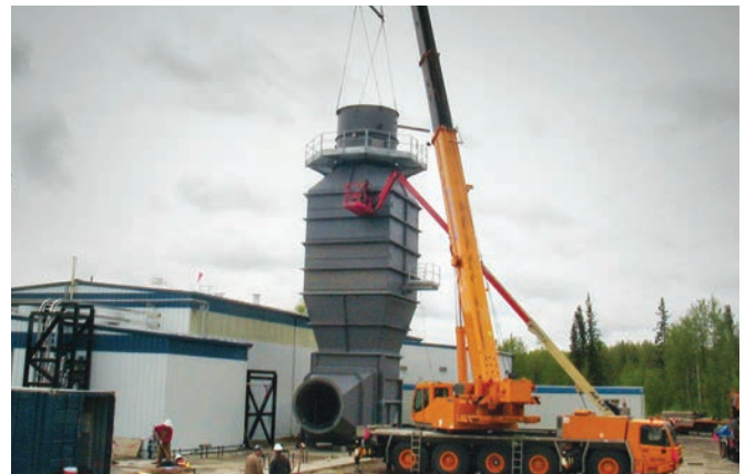
EXHAUST SYSTEM RETROFIT
