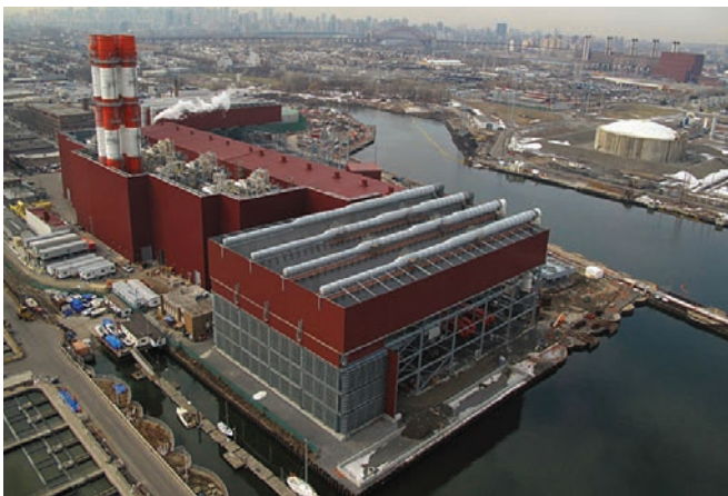
1000 MW ASTORIA ENERGY POWER PLANT, QUEENS, NY
