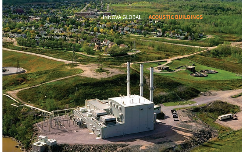
110 MW IROQUOIS FALLS COGENERATION STATION, IROQUOIS FALLS, ON
