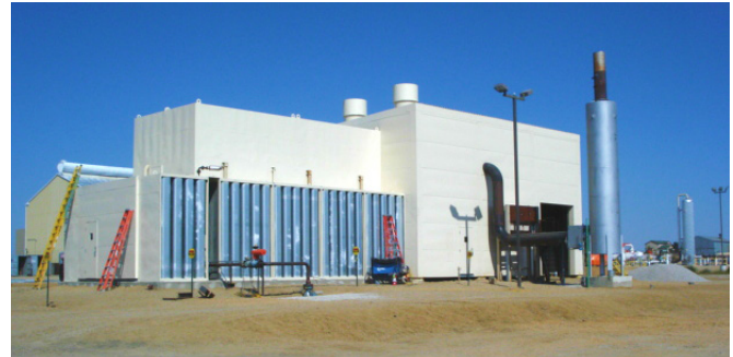
ACOUSTIC ENCLOSURE FOR A COMPRESSOR STATION IN FREDERICK, CO
